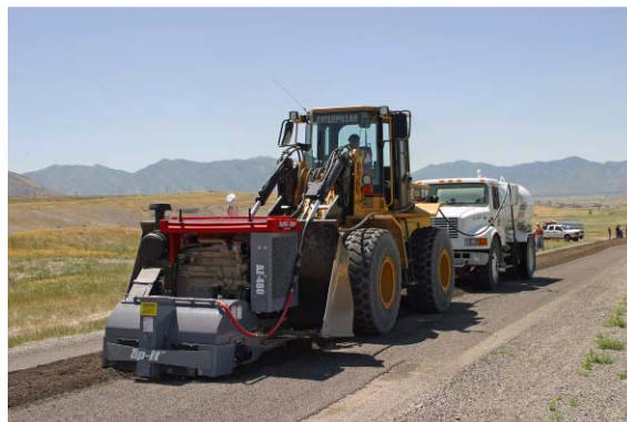
Figure 76. Photo. Equipment-mounted recycler.
