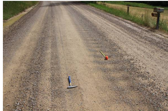
Figure 59. Photo. Chloride applied to poorly prepared road.
