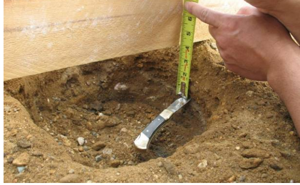
Figure 87. Photo. Checking gravel thickness.
