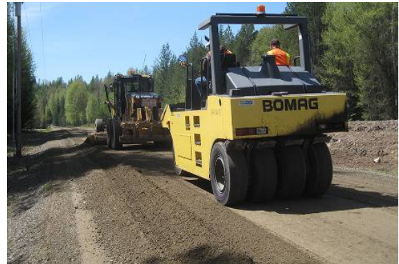
Figure 80. Photo. Compaction with rubber-tired roller.
