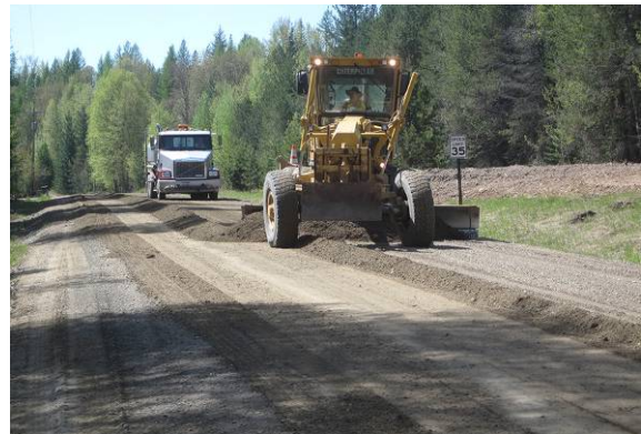
Figure 16. Photo. Maintenance of treated road.
