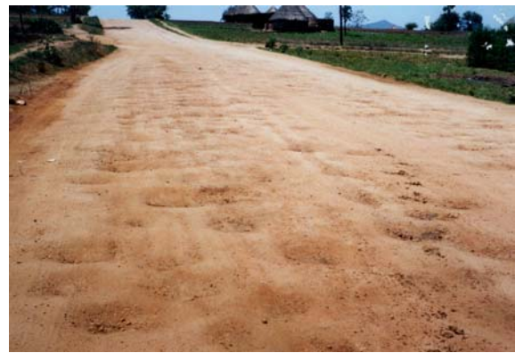
Figure 23. Photo. Potholes caused by poor drainage.
