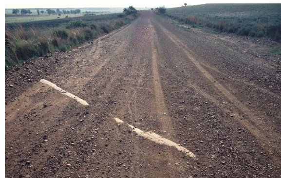
Figure 20. Photo. Insufficient, poor quality gravel.
