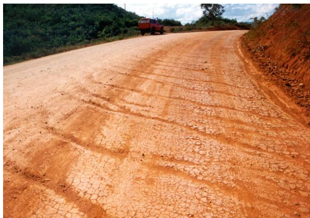
Figure 36. Photo. Transverse erosion.
