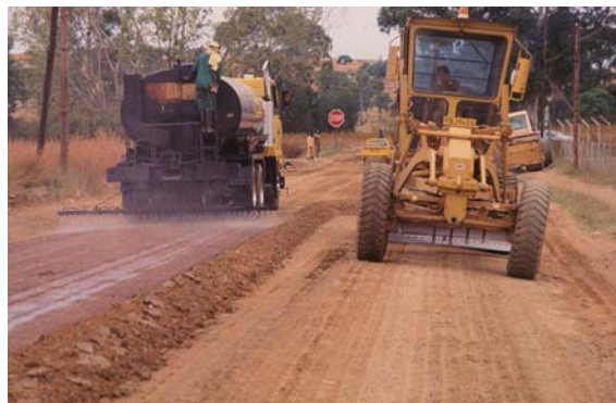
Figure 14. Photo. Mix-in treatment.
