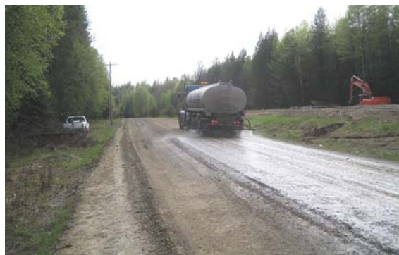
Figure 13. Photo. Spray-on treatment to well-prepared road.
