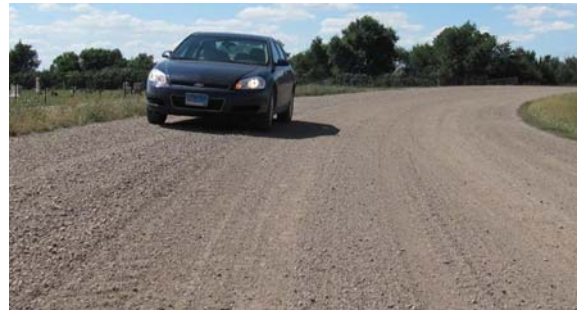
Figure 18. Photo. Super-elevation on sharp curve.
