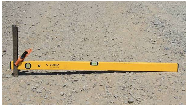
Figure 89. Photo. Checking crown with a simple level.
