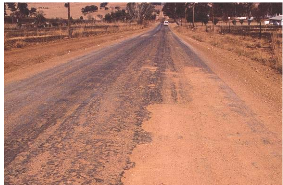
Figure 17. Photo. Broken crust.
