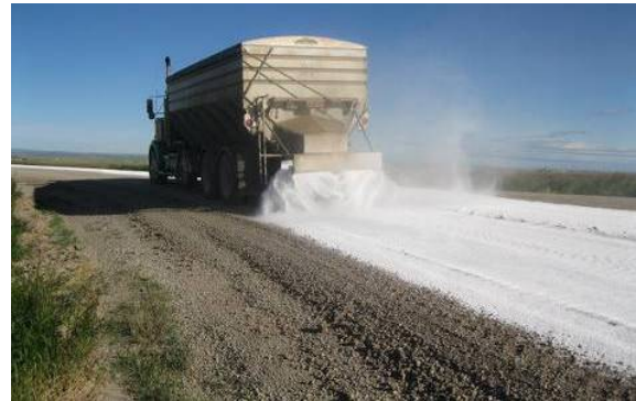
Figure 75. Photo. Flake application of calcium chloride.
