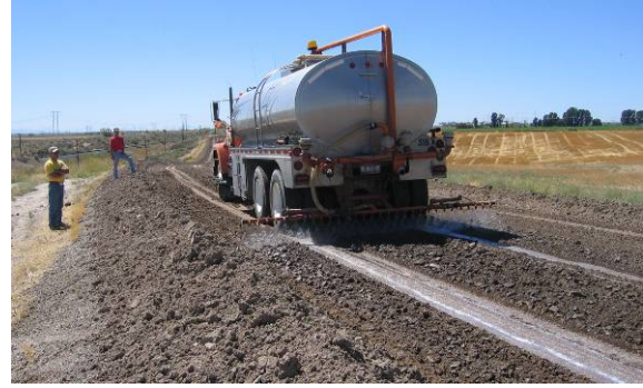
Figure 79. Photo. Spraying the additive.
