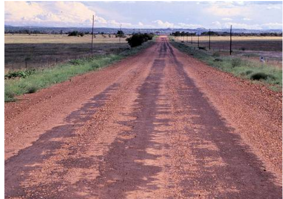
Figure 70. Photo. Insufficient additive application.
